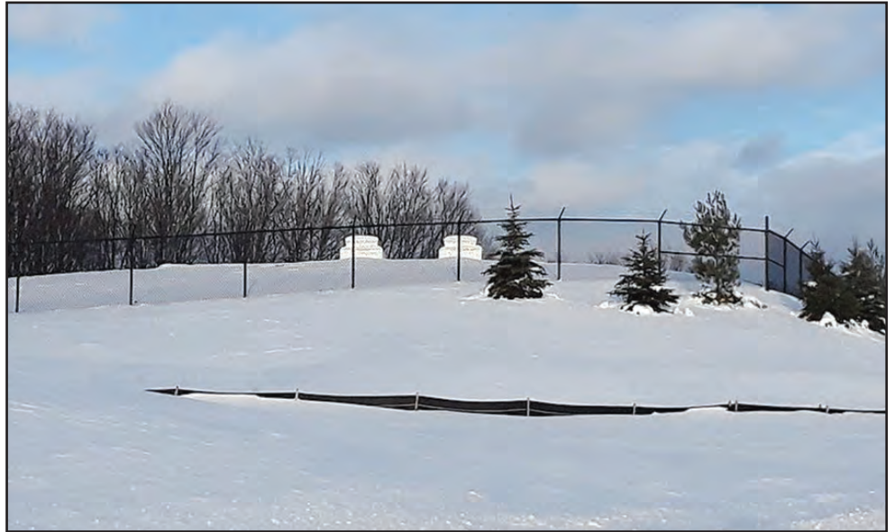
Finished storage tanks where the cement walls have been back-filled, the vents installed after the top was covered, and the area was fenced, and landscaped.
