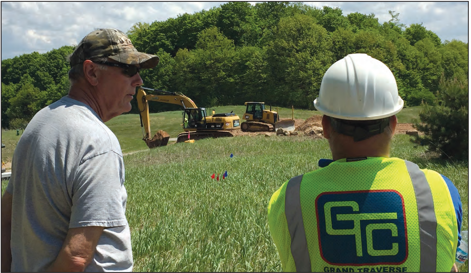
Steve Grill and a Grand Traverse Construction's employees inspecting the site adjacent to the Cedar River Well Field being prepared for the new in-ground storage tank.
