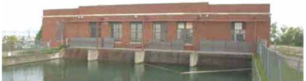
Elk Rapids Hydro Dam - view from upstream
