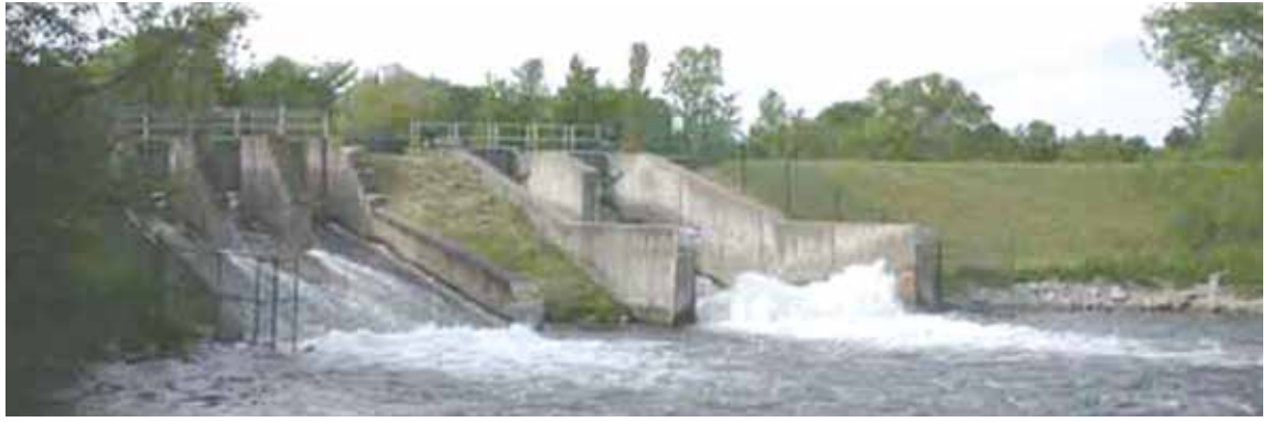
The Bellaire Dam - view from downstream
